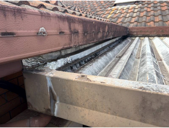
Patio skillion roof has been installed under house gutter.
